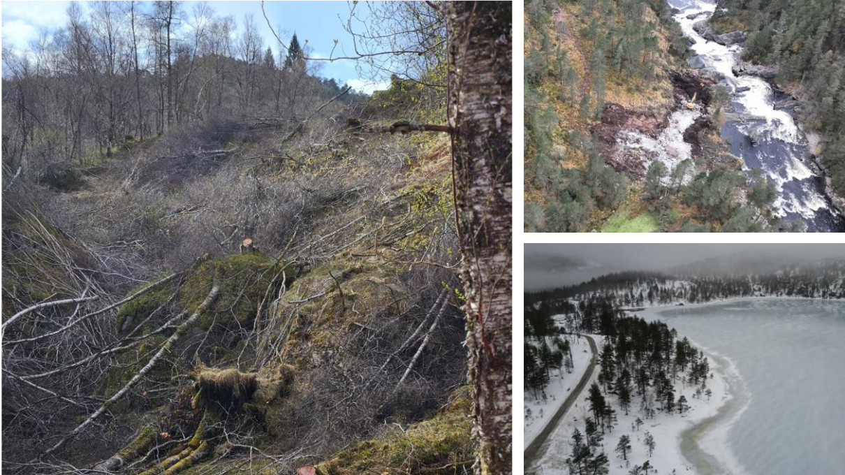
Different project. Smådalselva (big, left side), early startup, pipeline route. Frøytlandsfoss (up to the right), Intake area power station and Kjetevatn (down to the right), Flatland. Photo: Marianne B Kanstad and Alexandru Titi Georgescu
