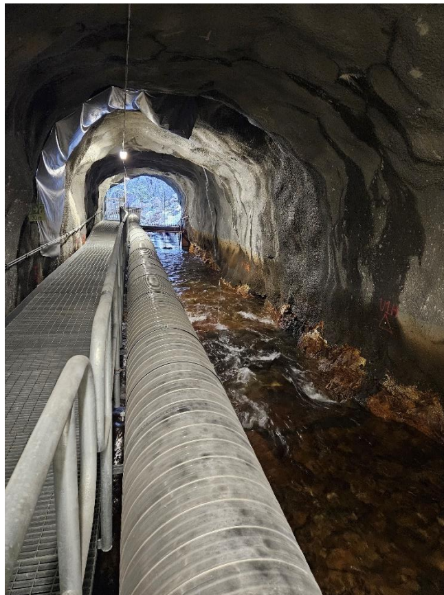
Holmen hydropower plant, water outlet, Atlantic salmon river downstream. Photo: Marianne B Kanstad
